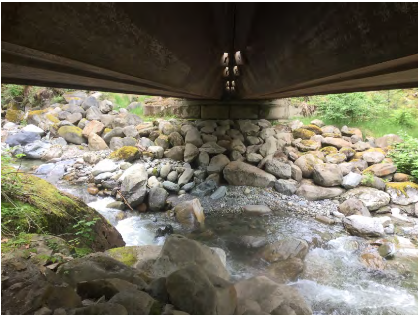
Left Bank Abutment when facing downstream
