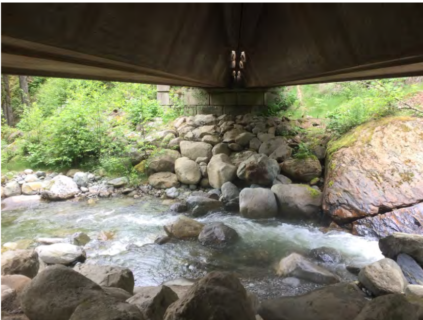
Right Bank Abutment when facing downstream
