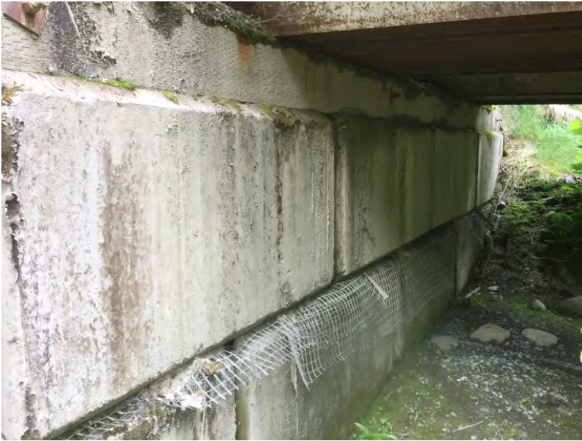
Right Bank Abutment when facing downstream
